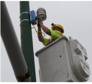
Array of Things: Cities are increasingly mounting sensors on buildings and street lights around the city to collect data about the environment, infrastructure, and citizen's activity to manage city issues such as climate, air quality, and noise. The sensors measure various data such as temperature, light, sound, and traffic. The real-time, location-based data that it collects is often available to the public.
